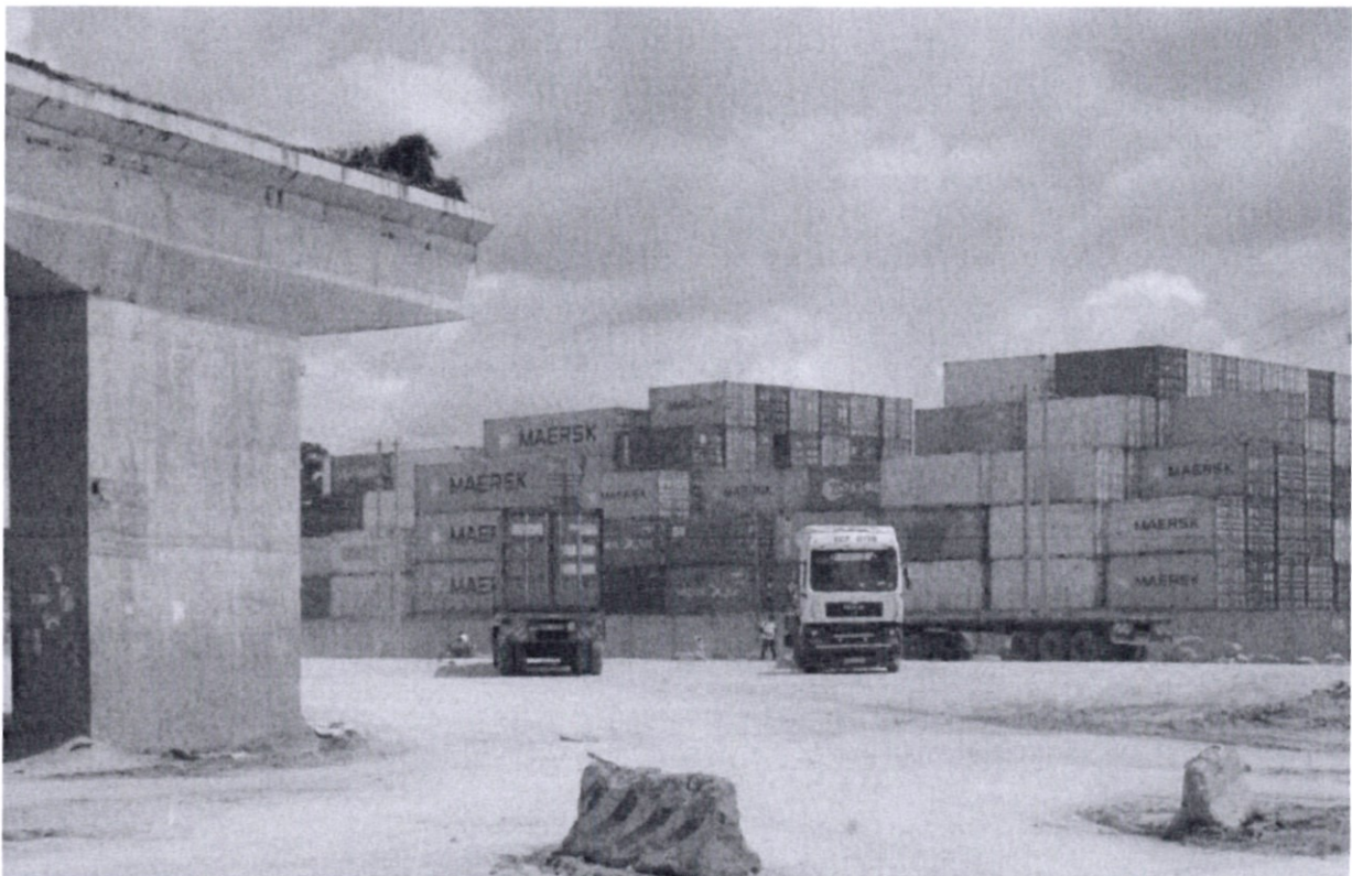
Figure 2: A section of the Mombasa-Mariakani Road undergoing construction.
