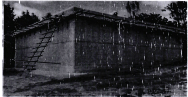
Figure 4: Chuka Water Supply Infrastructure-Ikuu Reinforced Concrete Tank
