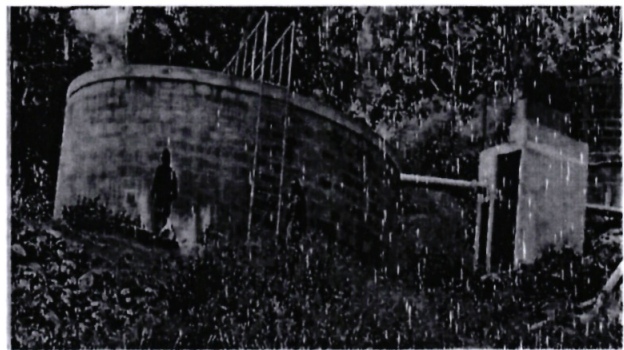
Figure 8: Marsabit Water Supply Infrastructure- Composite Filtration Unit
