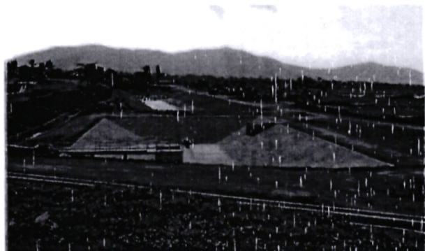
Figure 20: Chogoria Sewerage Infrastructure- Anaerobic Pond
