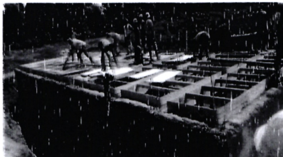
Figure 34: Kiawara DTF-Balancing Tank
