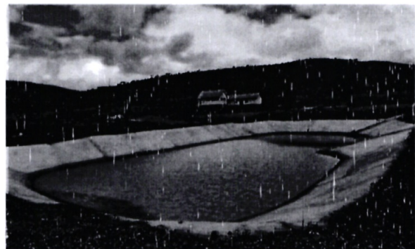
Figure 26: Marsabit Sewerage Infrastructure-Treatment Plant II
