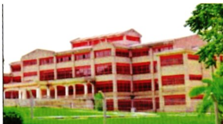
Ongoing construction of Library and Administration Block
