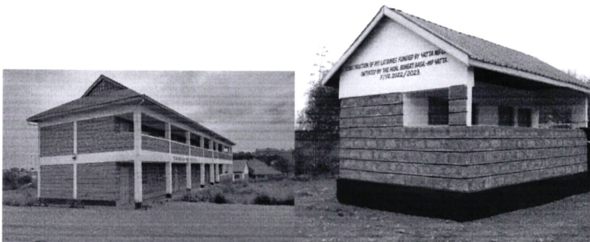
Katangi TTI-Construction of classrooms
