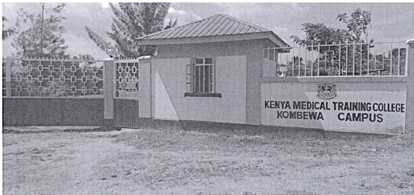
Figure 4: Construction of Morden Laboratory and 4 Classrooms
