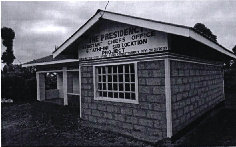
GITATHIINI CHIEFS OFFICE-CONSTRUCTION OF AN OFFICE BLOCK
