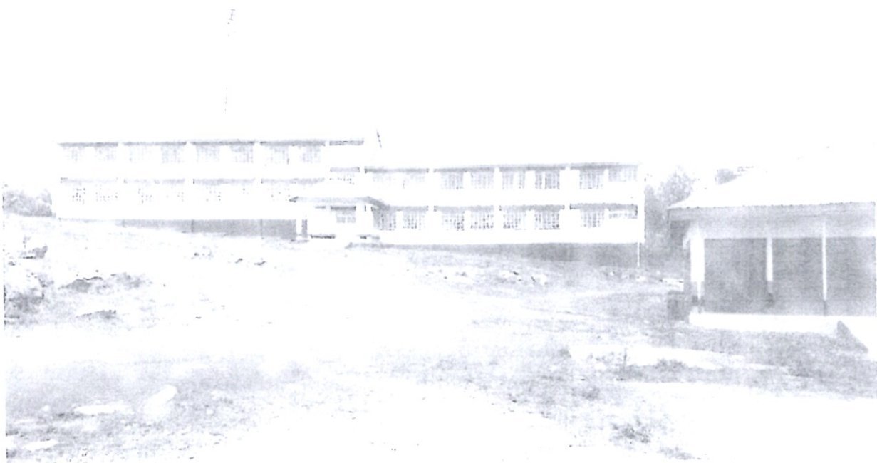
KMTC Navakholo – Construction of Storey building of 12 lecture halls in Bunyala Central Ward, complete and handed over
