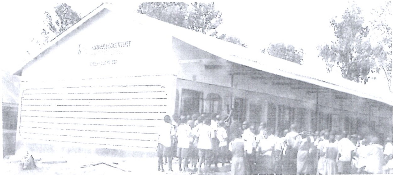
Kisembe Primary School – construction of 4no. classrooms in Bunyala West Ward, complete and handed over
