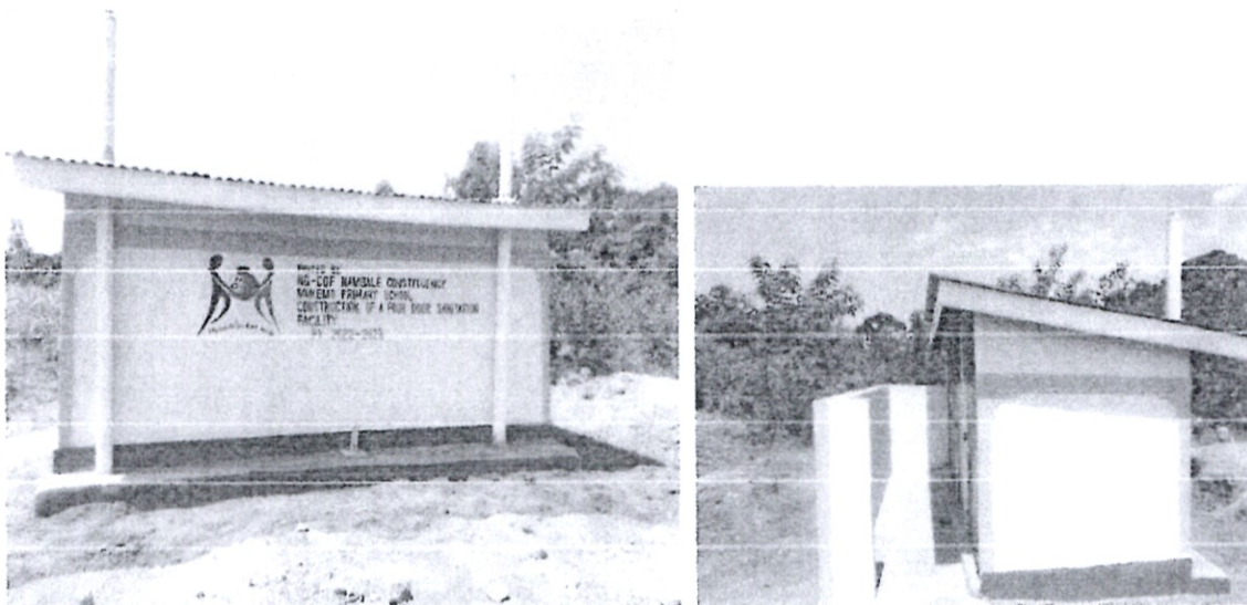
Fig; St. Peter Mukemo Primary school-construction of Four seater sanitation facility
