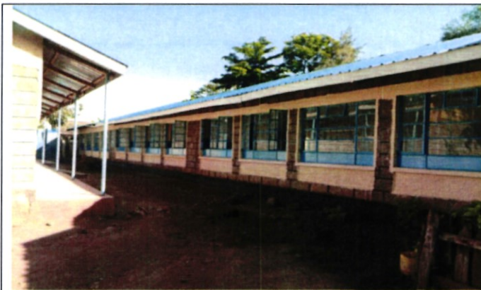
KoinangePri School - Renovation of 3 classrooms – Funded under emergency(Complete and in use)
