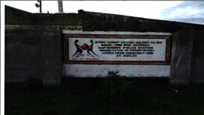
Kaptembwo Police Station - Rehabilitation of Perimeter wall – Funded under emergency(Complete and in use)
