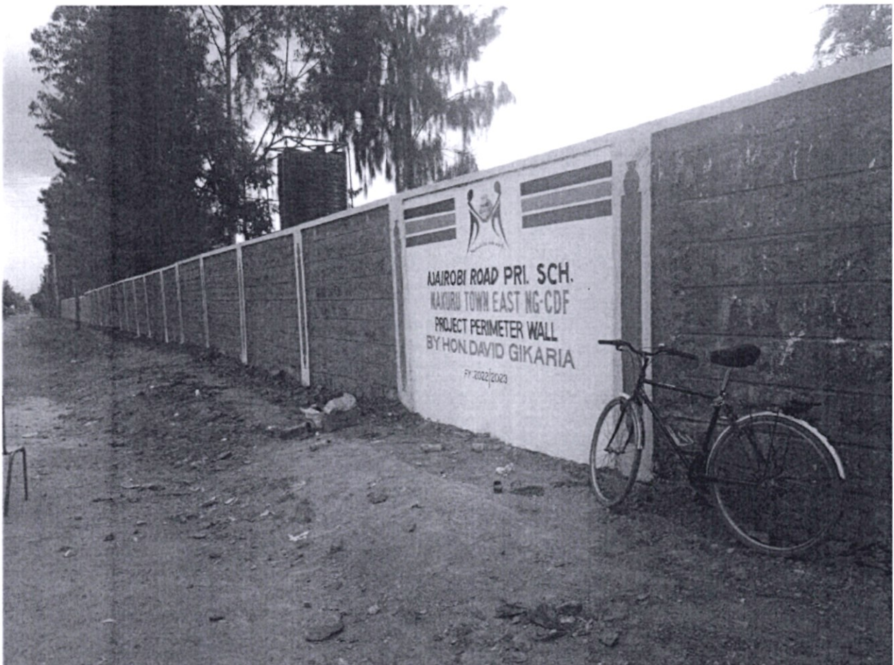
NAIROBI ROAD PRIMARY SCHOOL PERIMETER WALL
