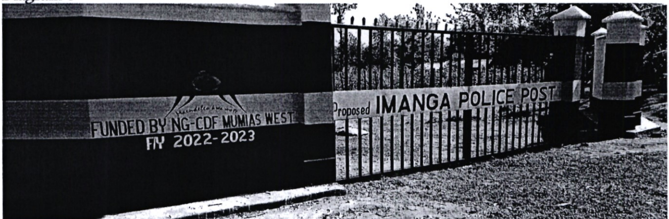
Imanga Police Post- Construction of Gate and fence.
