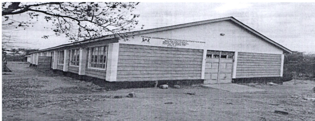
FIG 4: Mbuvo Secondary School-Dormitory
