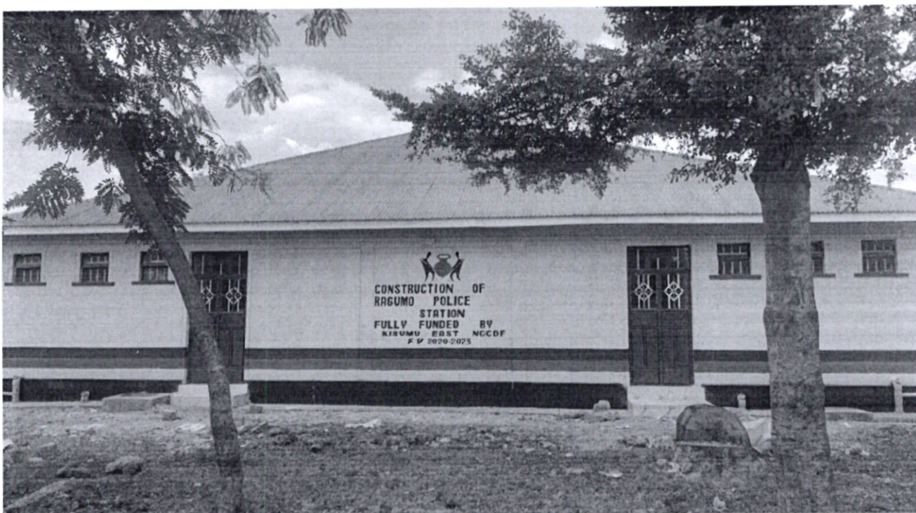
4.construction of ragumo police station
