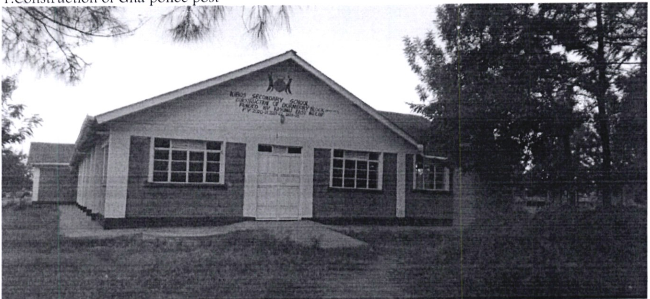
2. construction of a dormitory block at kibos secondary school
