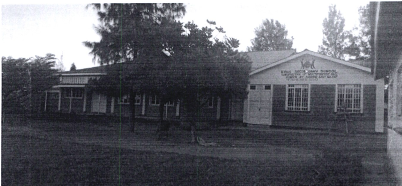
3.construction of a multipurpose hall at kibos secondary school
