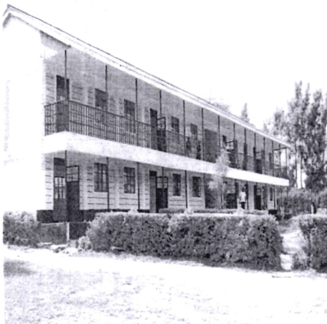
Nasianda Primary School (8 Classrooms storey)
