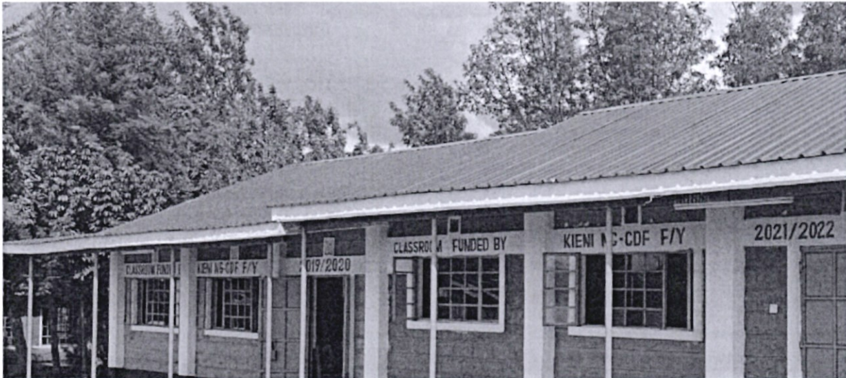
MWIYOGO PRIMARY SCHOOL CLASSROOM CONSTRUCTION
