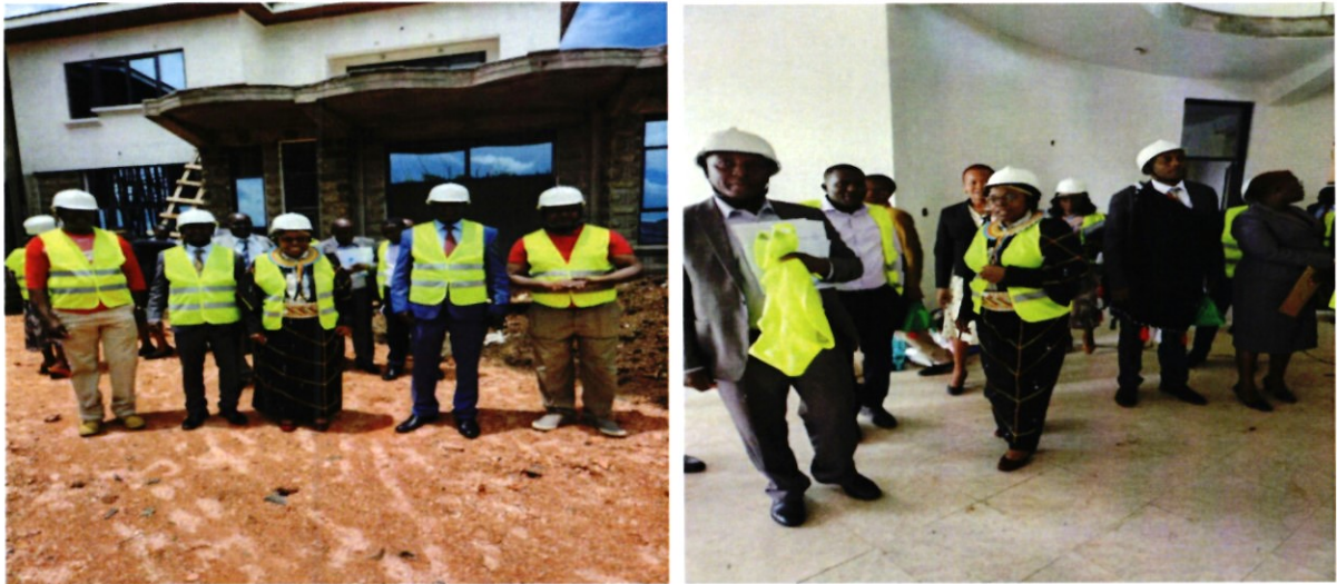
Figure 2: Construction of the West Pokot Governor's Residence
