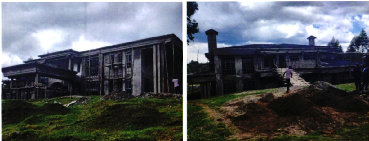
Figure 3: Ongoing construction of Kericho County Speaker's Residence
