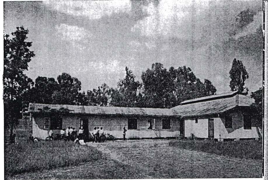
This building in Whitehouse Road, Nairobi was the first meeting place of Kenya's Legislative Council in 1907
