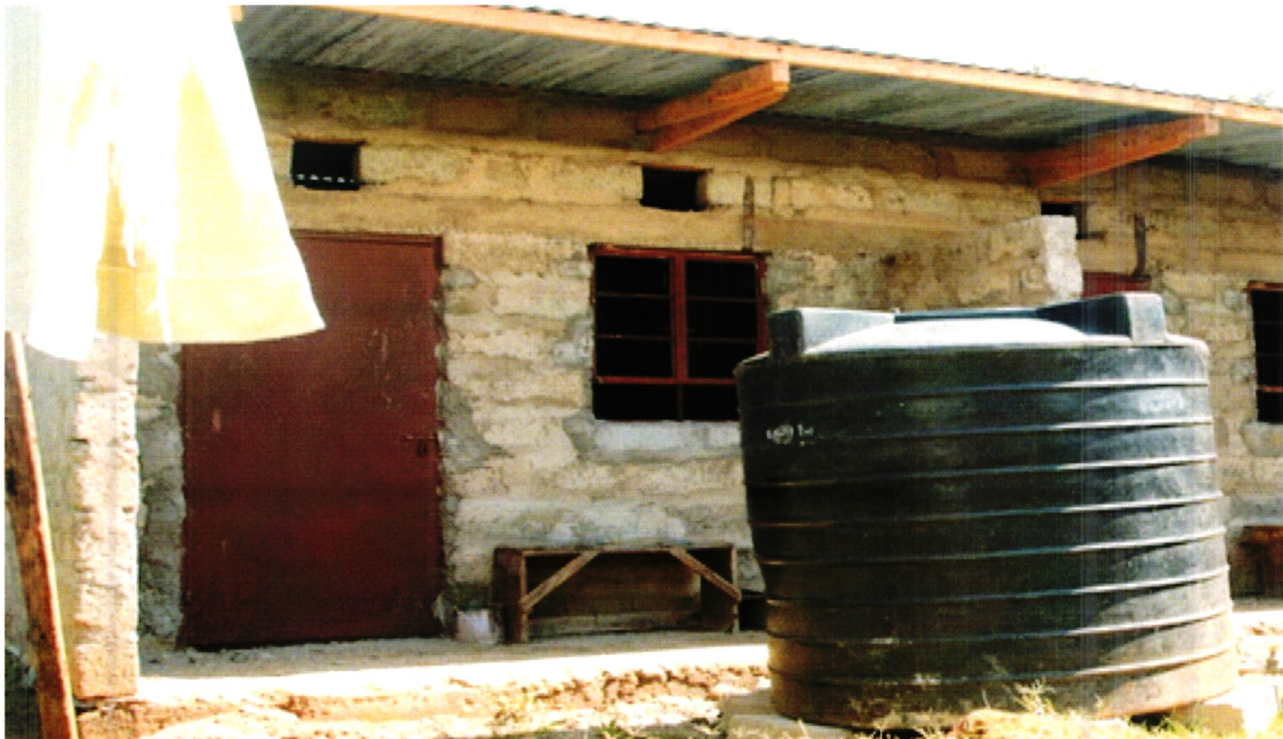
Tuuti AP camp houses constructed with support from Kibabii University to enable provision of security to students and the Kibabii University community.
