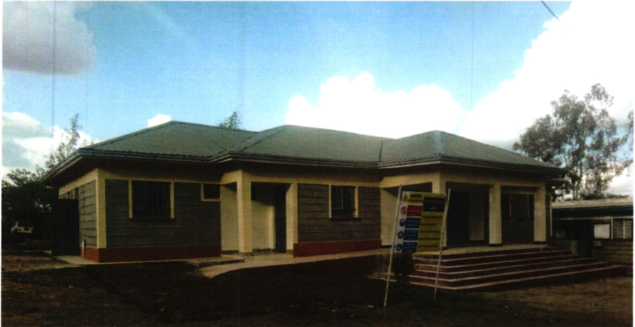
Newly constructed Samburu Office
