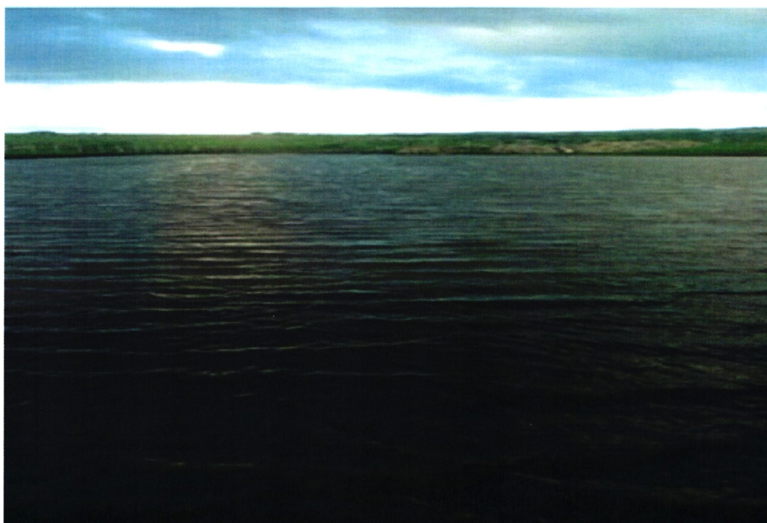
Oloyiungalani dam full to capacity
