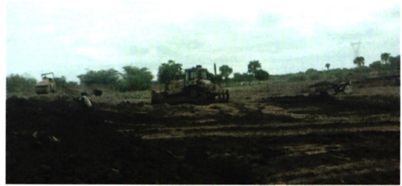
Repairs of the flood protection dyke section in at Mitapani breach at the preliminary stages
