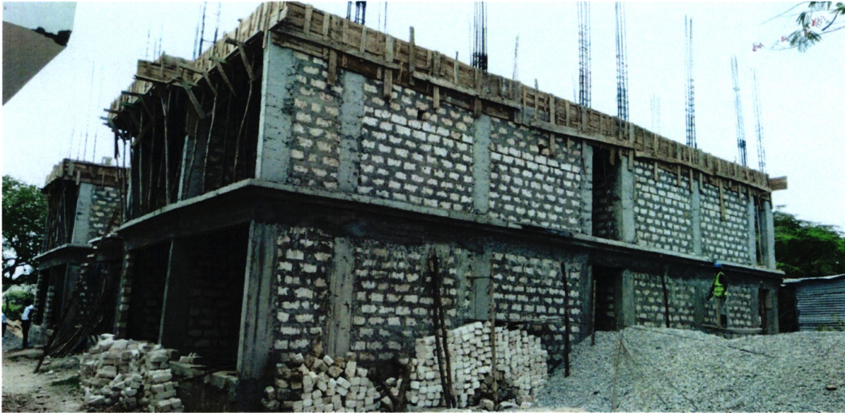
Construction of accommodation room in progress
