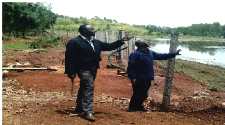
Overview of the Sama Mariki project showing the reservoir, fence and irrigation pipeline
