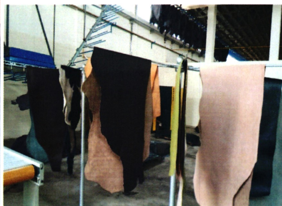
Installed overhead dryer
