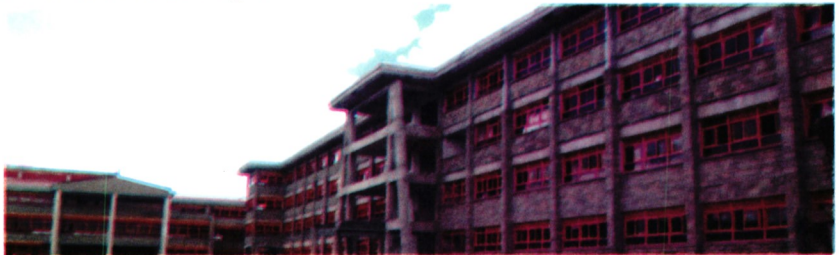
On-going Tuition Block and Library & Administration Projects
