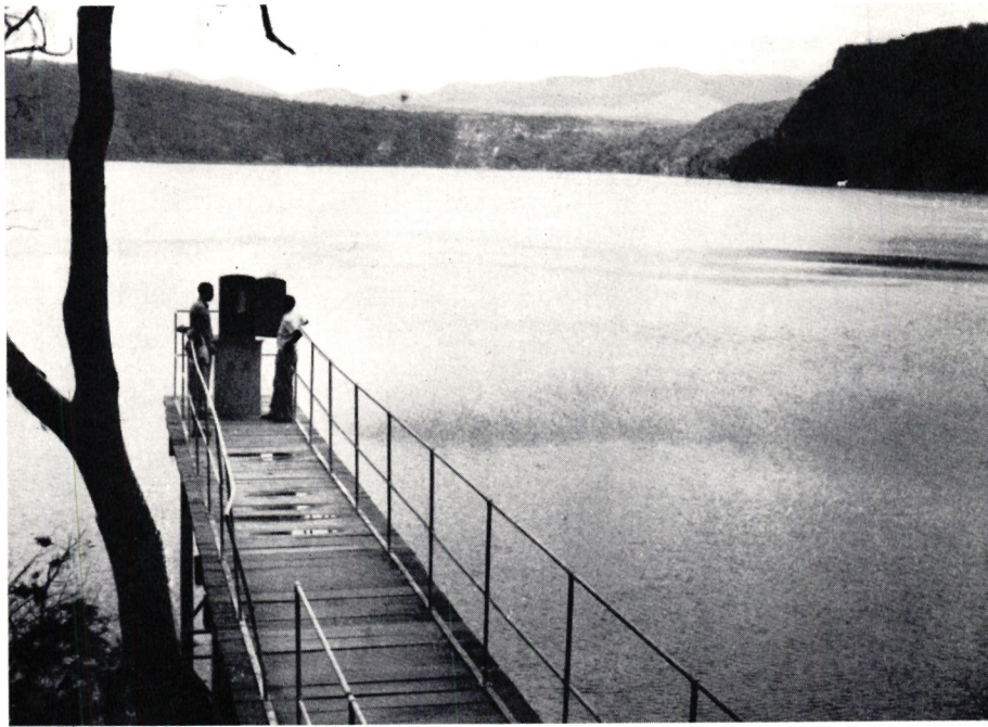
Fig. 5.—The Regular Gauging Station on Lake Chala showing the Water Level Recorder.
