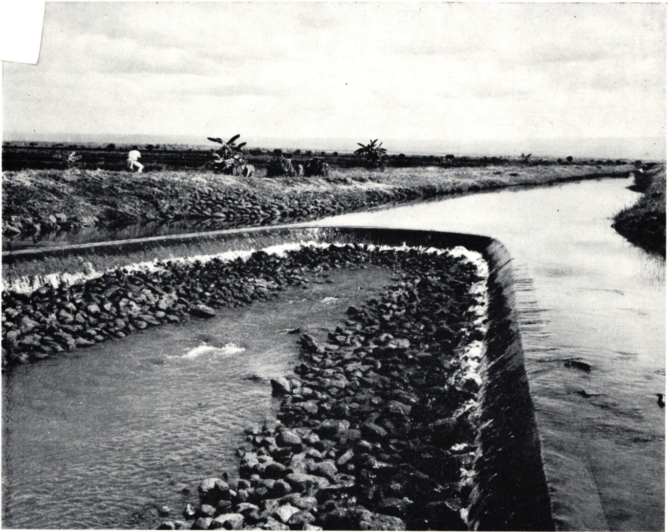
Fig. 7.—MWEA IRRIGATION SCHEME.—Long Crest “Horseshoe” Weir giving Minimum Level Variation with Full Flow Range. (Flow Range 0–150 cusecs: level variation 0.45 feet.)
